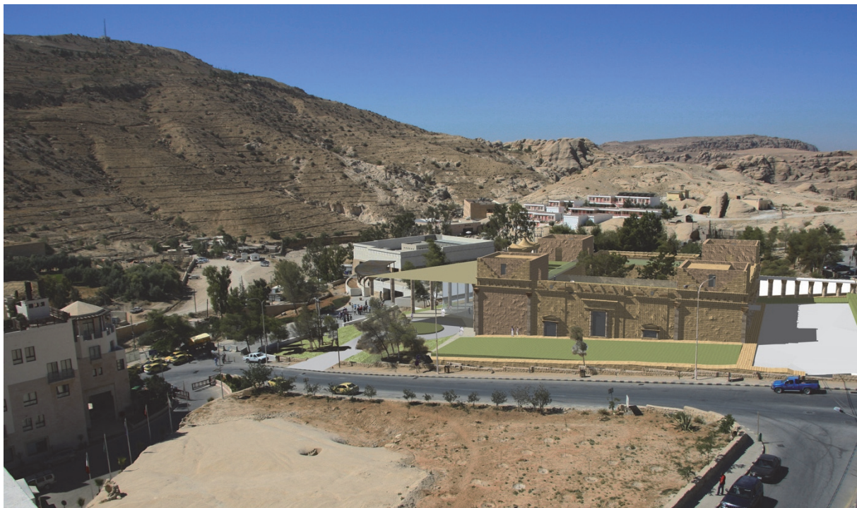
Viewpoint 9: From the Petra Moon Hotel's roof on the east side of the site The appearance is divided into small scale.
