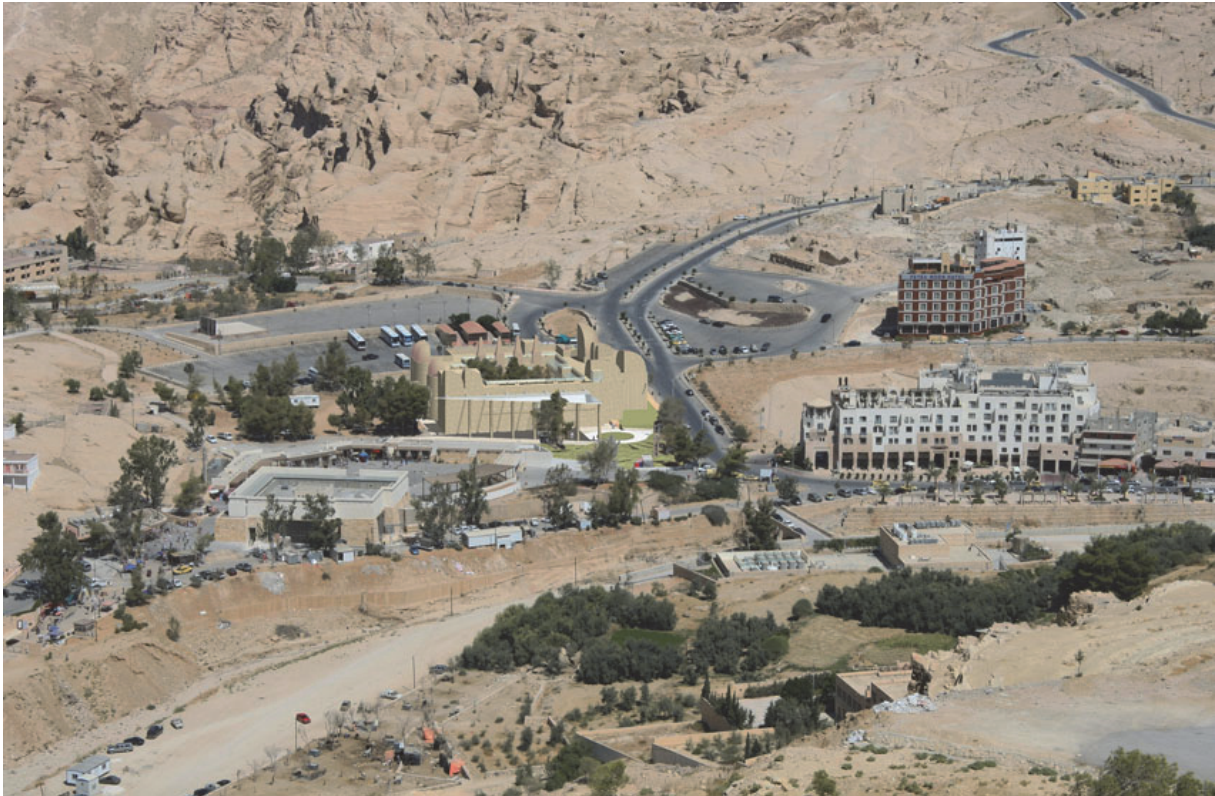
Viewpoint 1: From the roof of the PDTRA office The simple curved wall harmonizes with the landscape of the sandstone mountains.
