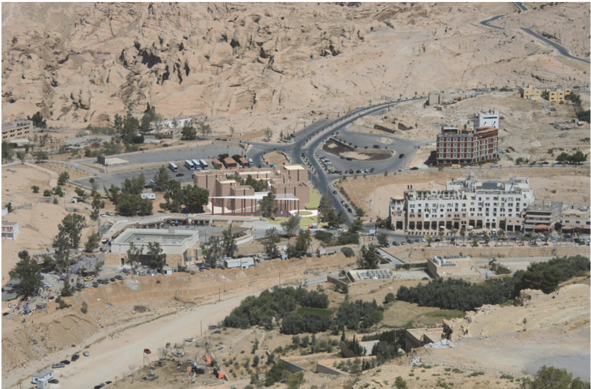
Viewpoint 1: From the roof of the PDTRA office Visitors can walk on the roof.
